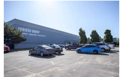
555 Conestoga Boulevard, Cambridge, ON
