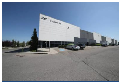
7007 54th Street SE (Building D), Calgary, AB
