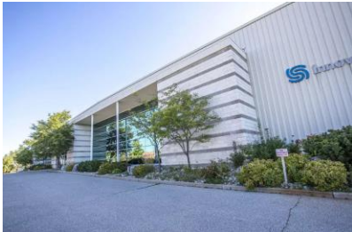
549 Conestoga Boulevard, Cambridge, ON
