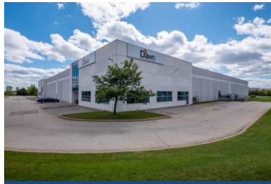
275 Steelwell Road, Brampton, ON
